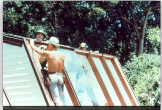
Figure 3. Hobby greenhouse being constructed with double glazed patio door glass.
