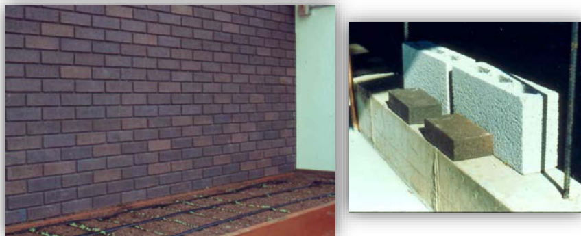
Figure 1. Brick storage wall in passive solar hobby greenhouse – Thermal storage mass is a wall made with two layers of brick filled with concrete. In this well-built structure, nighttime temperatures dropped to 35°F with no supplemental heat when outside temperatures dropped to -17°F. Note young crops in raised-bed style garden with drip irrigation.
